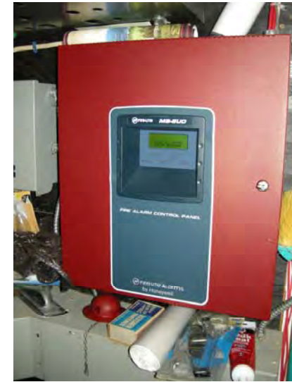
Fire alarm control panel
