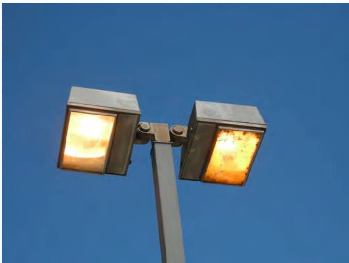
Double headed site lighting fixture
